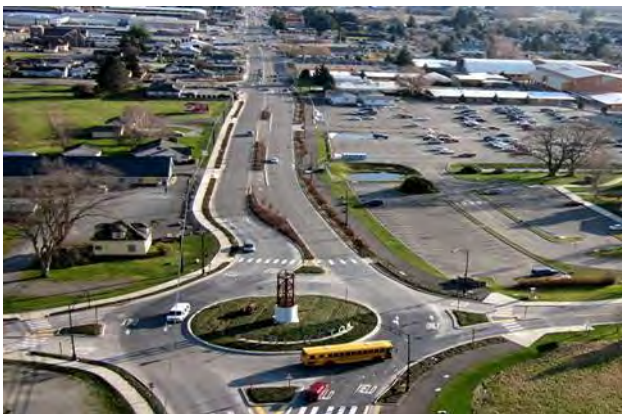
North Burlington Boulevard Roundabout
