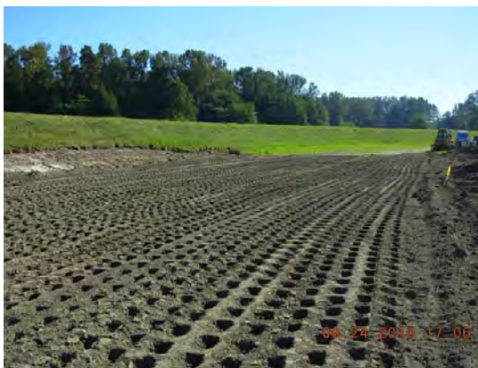
2010 Dike 12 levee work: NW quadrant, looking south
