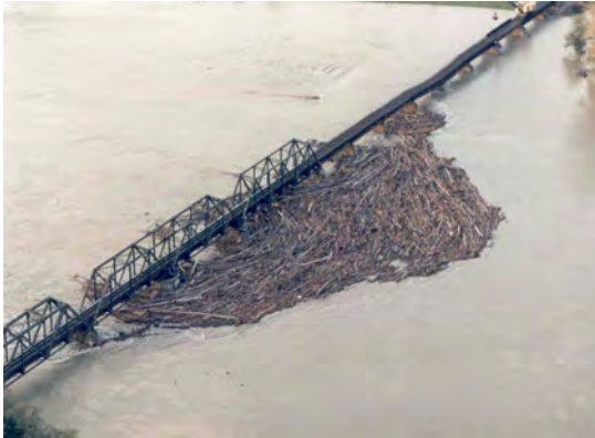
1995 Skagit River Flood – BNSF Bridge failure
